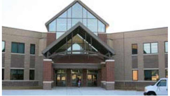
Manheim Township High School is an addition and renovation project for 1800 students of approximately 360,000 square feet.
